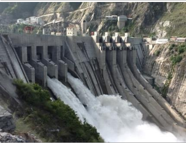
Hydro-Electric Power Station, Baglihar II, India
